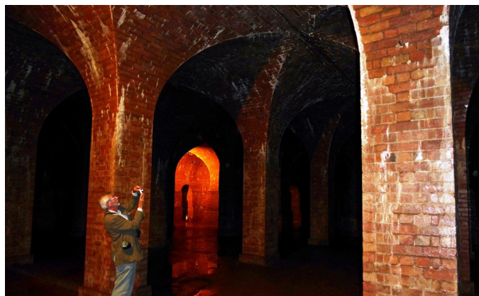
The underground reservoir at Papplewick
